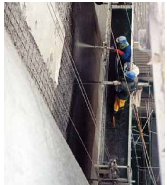
Fig. 3: Concrete spraying
