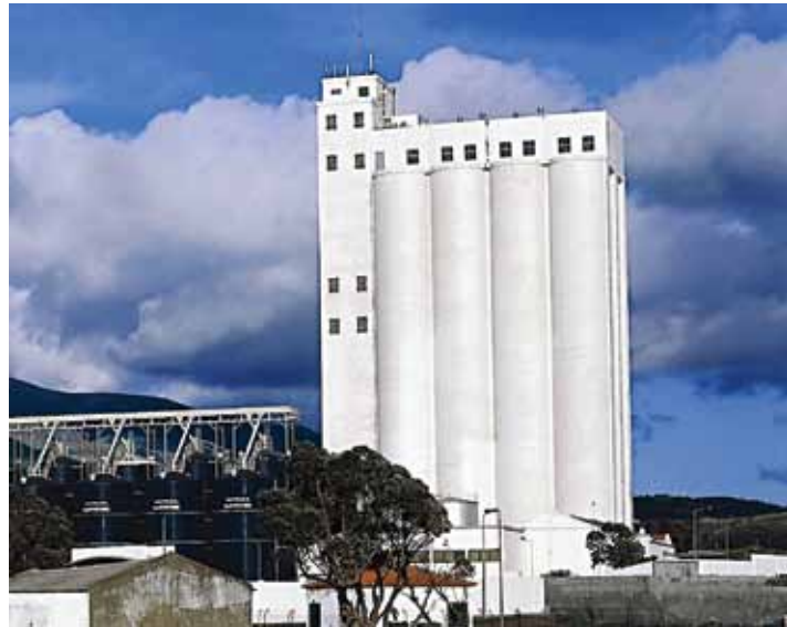
Fig. 5: Recent view of the rehabilitated Lagoa Silo
