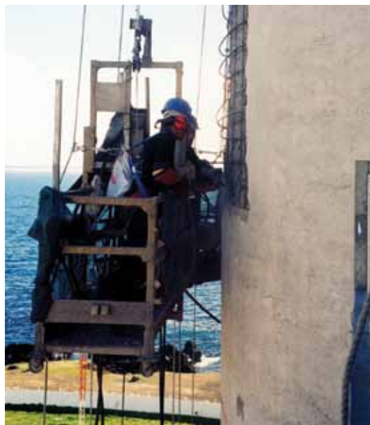
Fig. 2: Removal of deteriorated concrete
