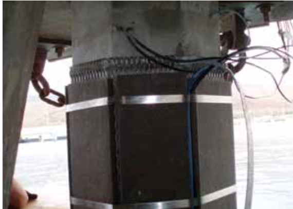
Zinc and compression panels installed and held in place with bands
