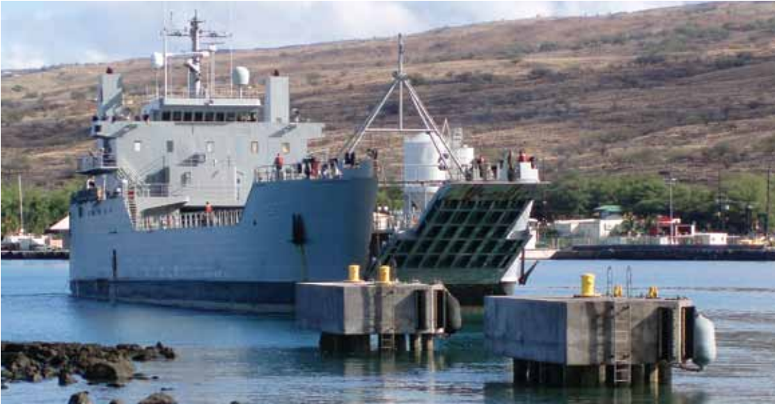
Mooring dolphins, built in 2001, are supported by prestressed, octagonal piles. The piles are driven directly into the bottom of the harbor sea floor
