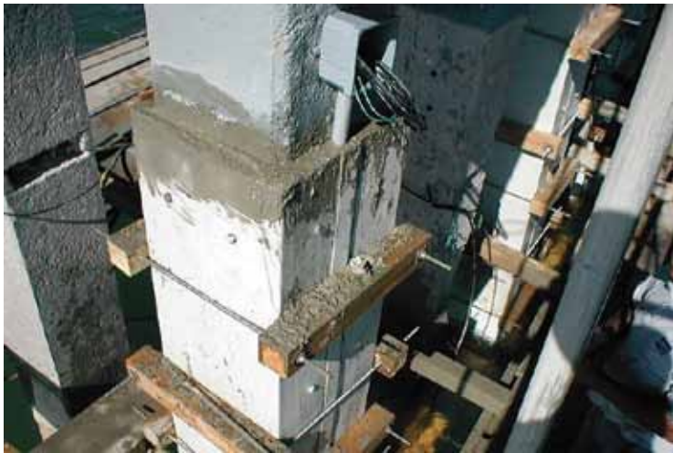
Lifejackets filled with concrete
