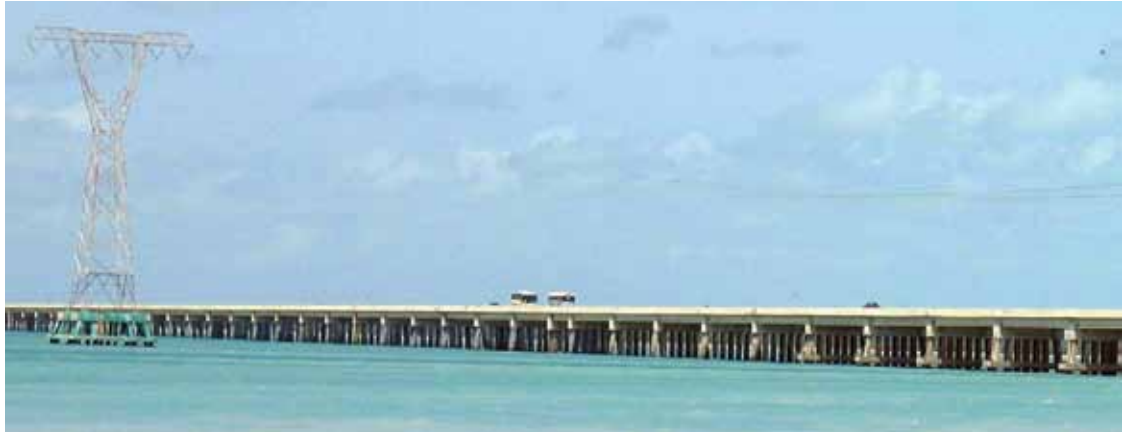
Overall view of the bridge structure
