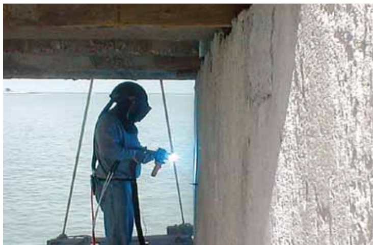
Metalizing bent caps
