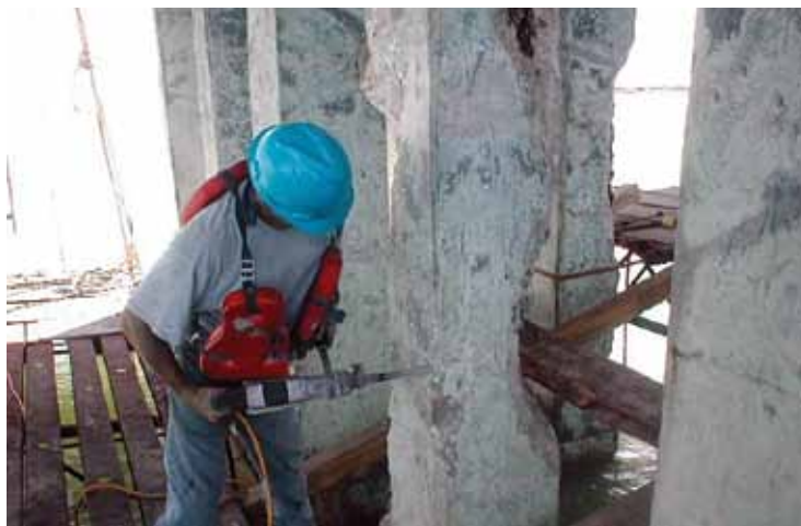
Removal of deteriorated concrete
