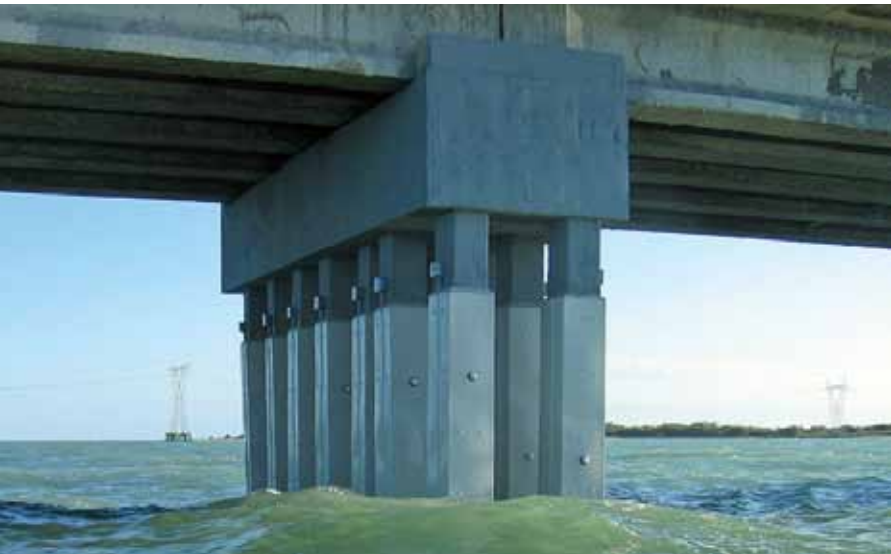
Completed cathodic protection system on bridge piles and bent cap
