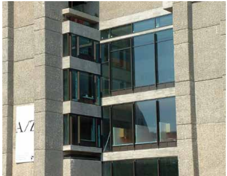
East façade after concrete rehabilitation and window replacement
