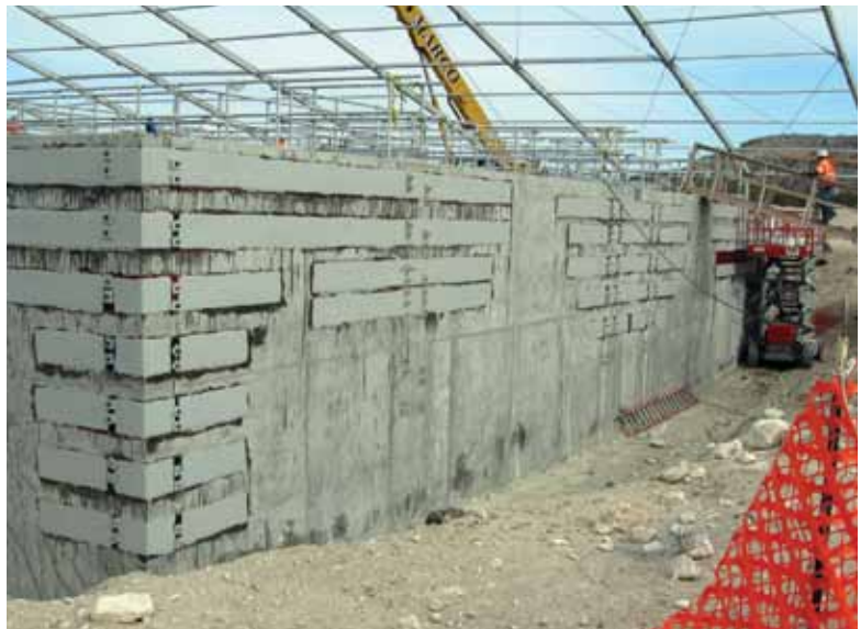
External corner of structure showing CFRP, anchorage, and temporary tent erection
