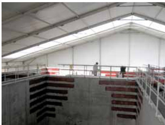
Ambient winter conditions required temporary heat and tenting of entire structure
