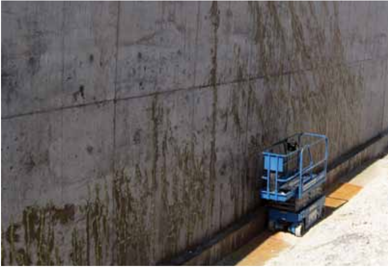
High-pressure epoxy injection of cracking
