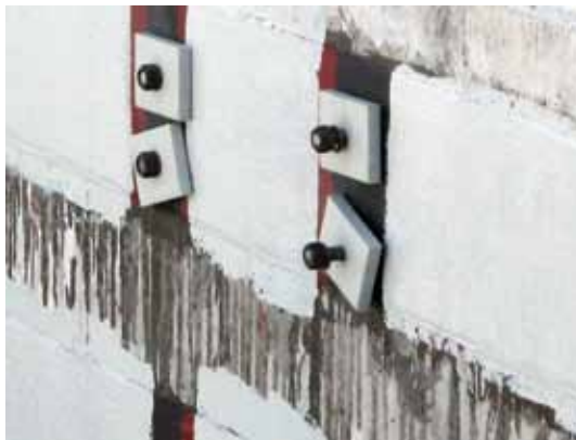
Bolts and plates at wall intersection (opposite side of wall pictured)
