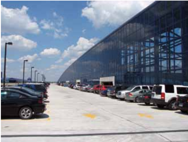
Detroit Metropolitan Airport Blue Deck Parking Structure
