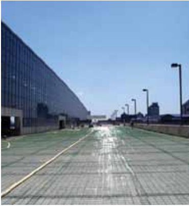
Roof deck with reinforcement in place and overlay to be installed
