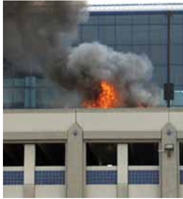
Car fire on the roof of the repaired structure in November 2006
