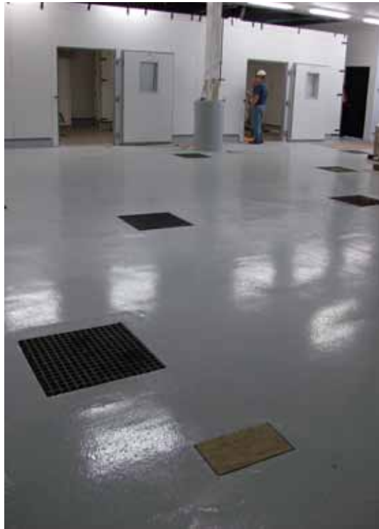
Completing lab finishes
