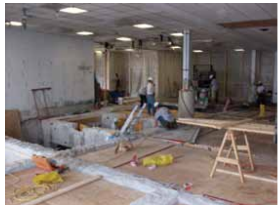
Demolition and forming
