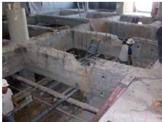
Demolition at Wet Lab A
