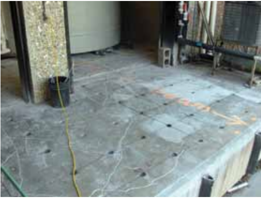
Cored holes and slots for galvanic protection
