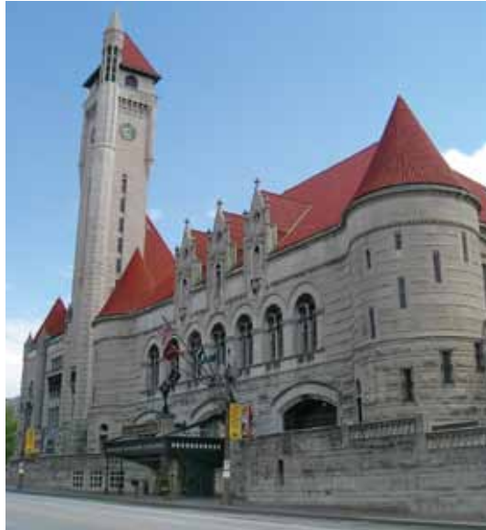
Fig. 1: Market Street façade of the St. Louis Union Station Headhouse
