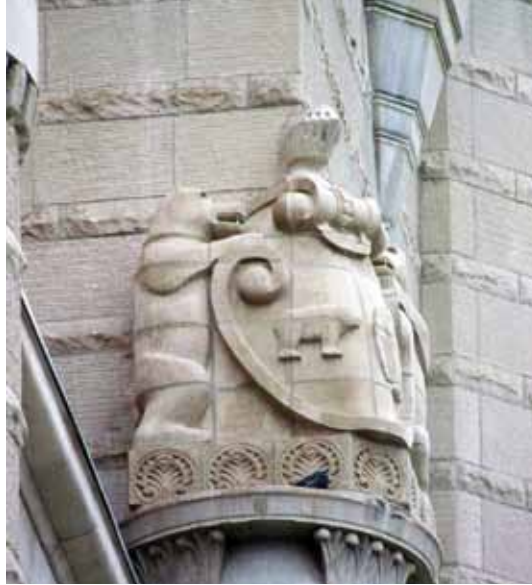
Fig. 6: Installation of the replacement crest is nearly complete
