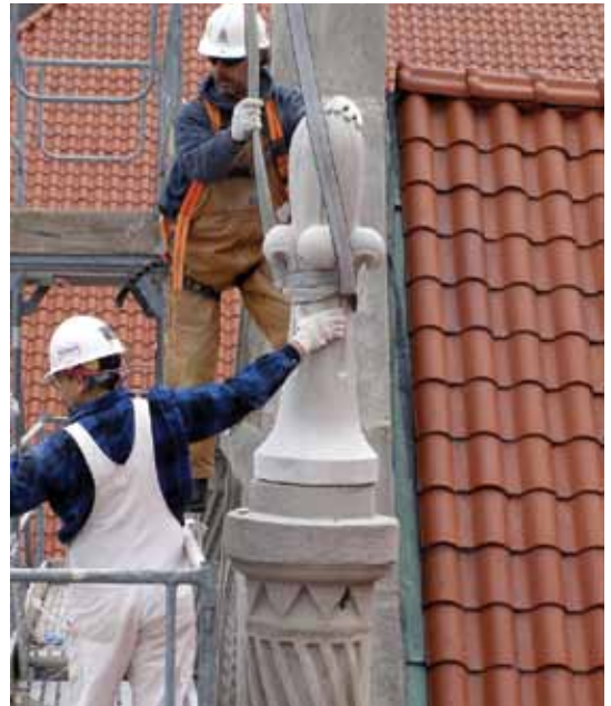
Fig. 4: Installation of new limestone finials to match the originals
