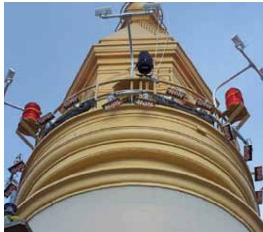
Fiberglass-reinforced polyurethane liquid-applied membrane in custom gold to match the original
