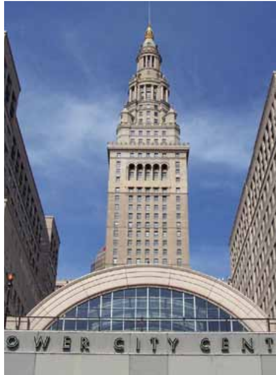
Terminal Tower Façade Repair Project, Cleveland, OH
