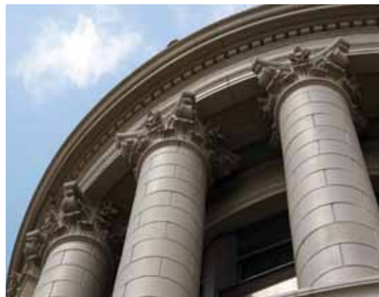
A total of 32 fiberglass columns replaced the originals
