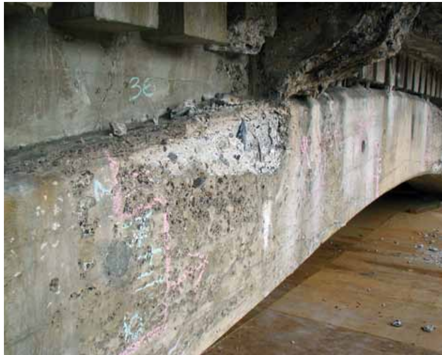
Arch deterioration
