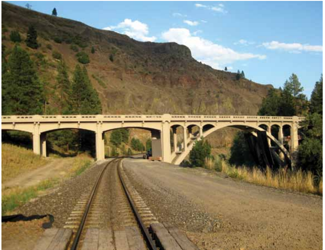
Upper Perry Arch Bridge after restoration
