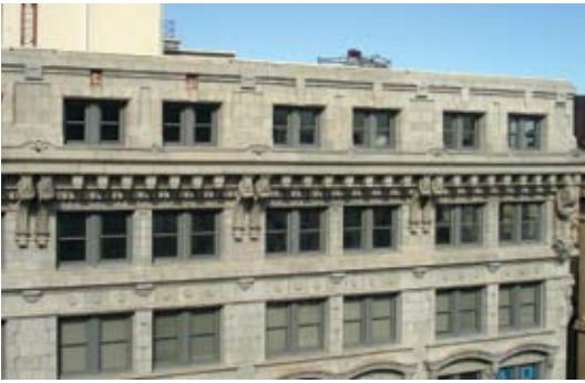
Completed FRP cornice
