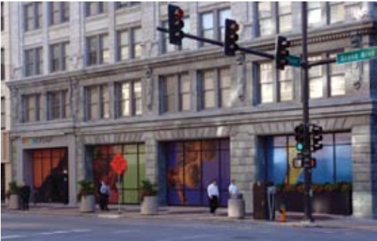
Front entry after completion
