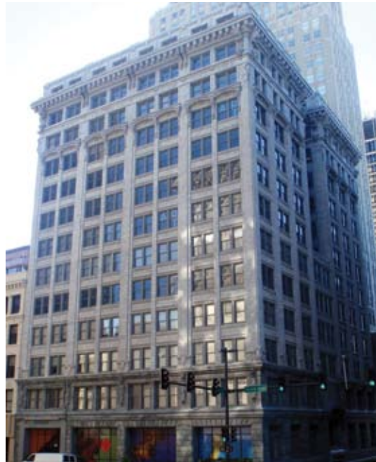
Completed project after repairs
