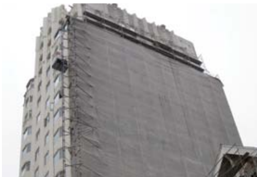
Twenty-story scaffolding erected on the west wall, fully enclosed
