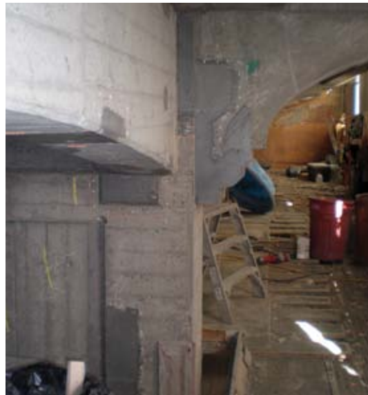
More complex, three-dimensional repairs can also be completed with the solution created by the team. Forming and pumping does not limit the repair to flat surfaces. Note the architectural corbel formed just right of center. Remnants of the white plastic tapit shells are still in the wall, used to hold the form in place
