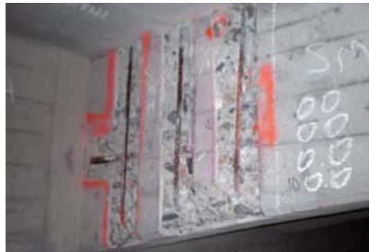
The repair has been prepared. Rather than cutting out reinforcing bar, the surrounding concrete is prepared and a box form will be built around it
