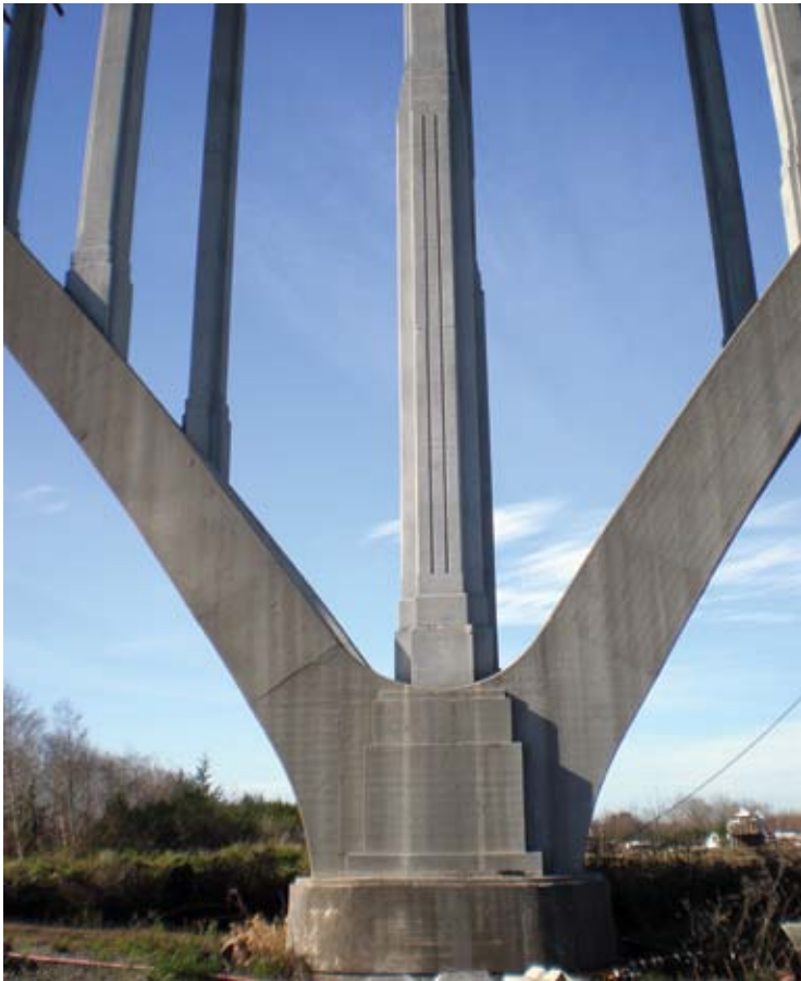
Inside the enclosure you could see the series of platforms that reached out to the center of the enclosure, which was currently erected around one of the main support columns. This photo shows the graceful sweeping nature of the design of this bridge. Note how the arches come together from either side to meet the column. The surface of the repairs has been sandblasted and coated with zinc as a part of the cathodic protection system
