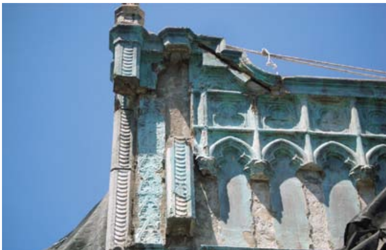
Demolition to remove unsound concrete
