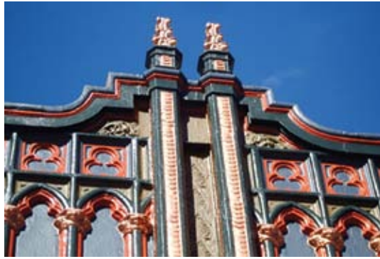
Close-up of completed repair
