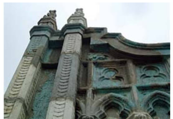
Freehand work to repair unsound concrete and match existing units
