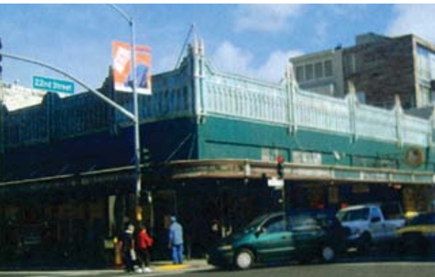
Project before repair work
