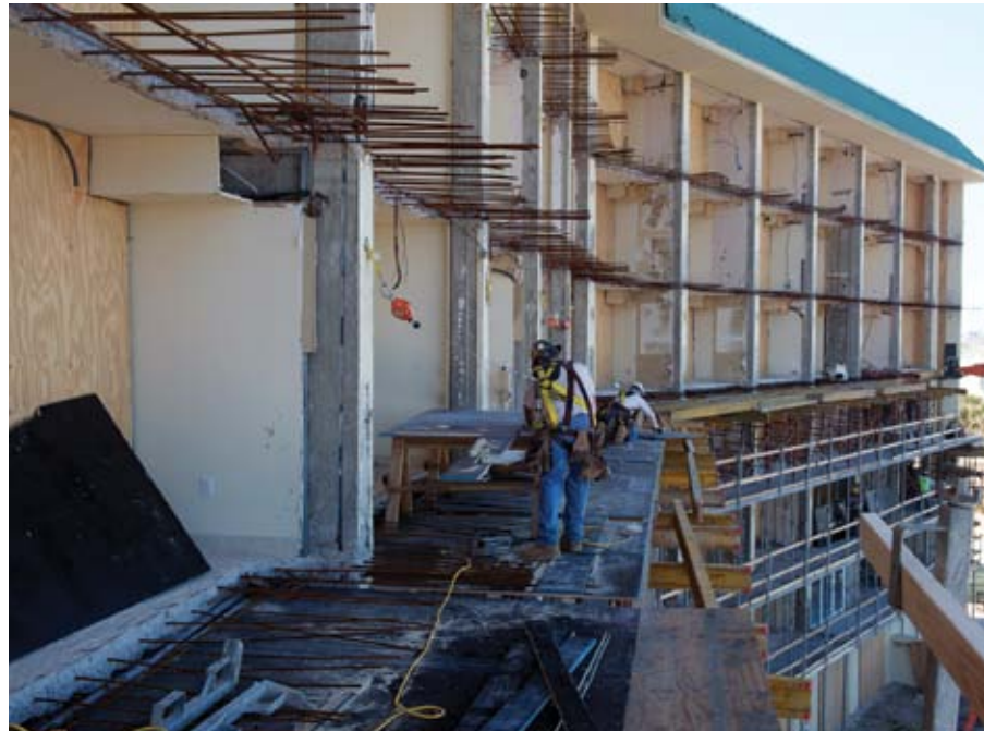
Work proceeding on balconies
