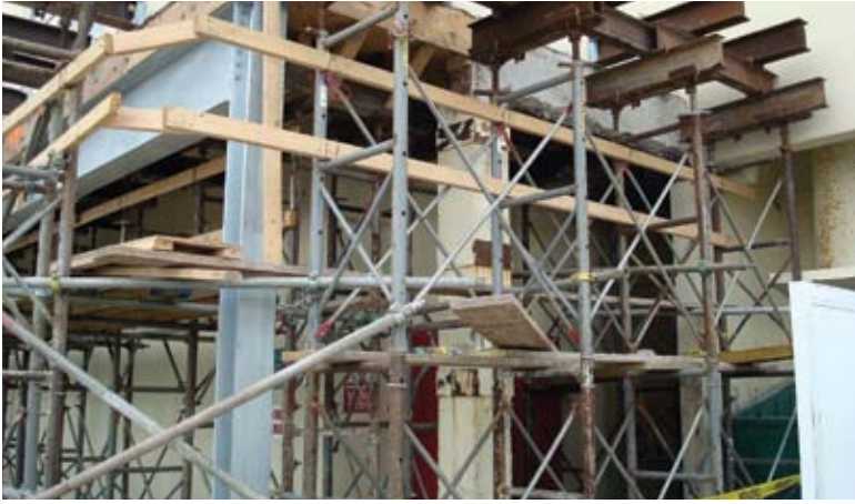
Replacement structural steel columns and beams
