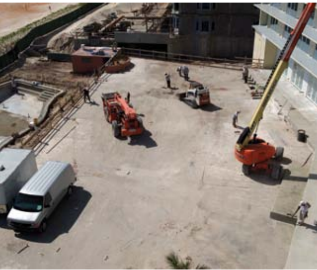
Work proceeding on new deck and pool area
