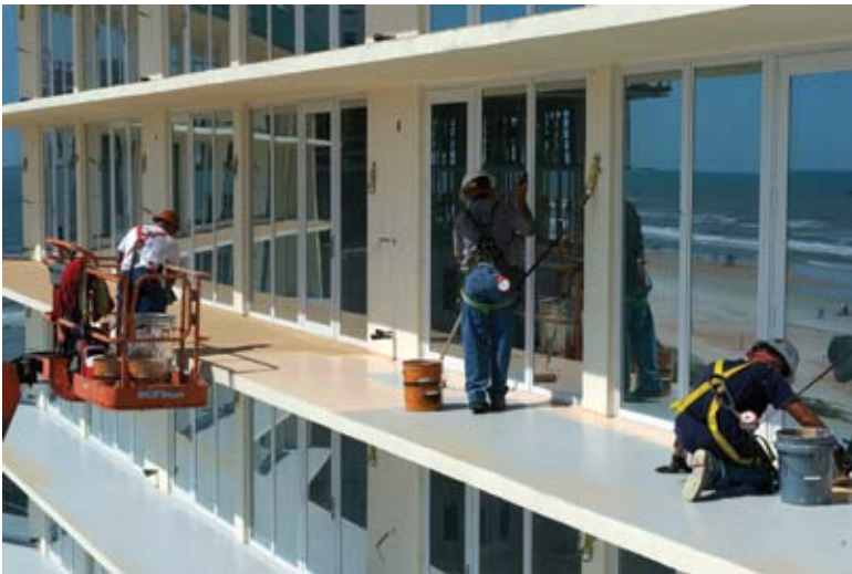
Coating being applied to new balconies
