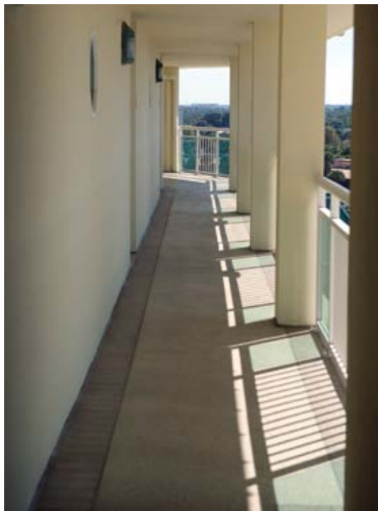
Finished balcony with new railing
