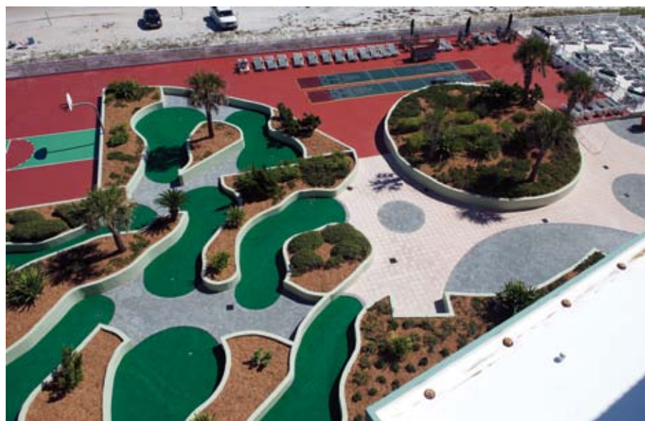
New recreation deck area
