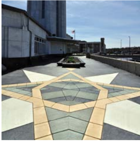
Overall view of completed integrally colored design feature in the concrete plaza slab
