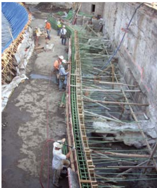
Rebuilding the concrete fishing platform using epoxy-coated steel reinforcement
