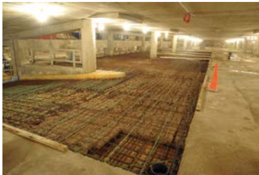
Prepared repair area with steel replacements
