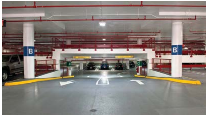
Completed parking garage interior
