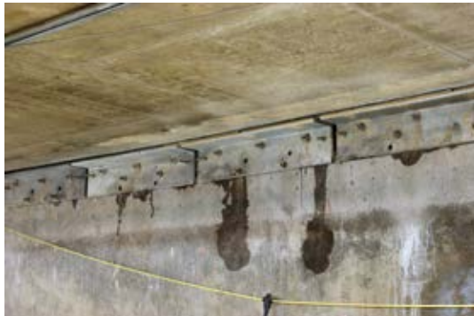
Installed steel support angles
