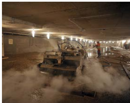
Hydrodemolition of deteriorated floor area
