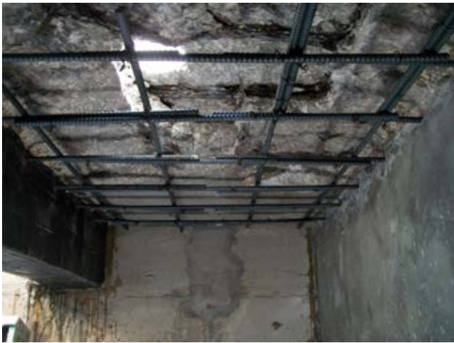
View of overhead deck area showing replaced reinforcing steel
