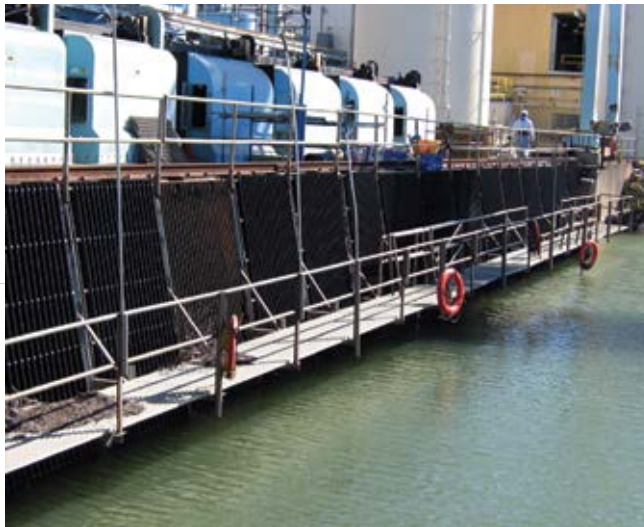
External view of intake structure
