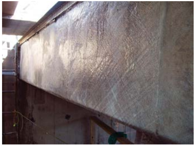
Fiber-reinforced polymers encasing existing beam
