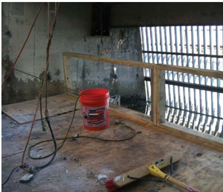
Floating platform fabricated to work inside intake chambers
