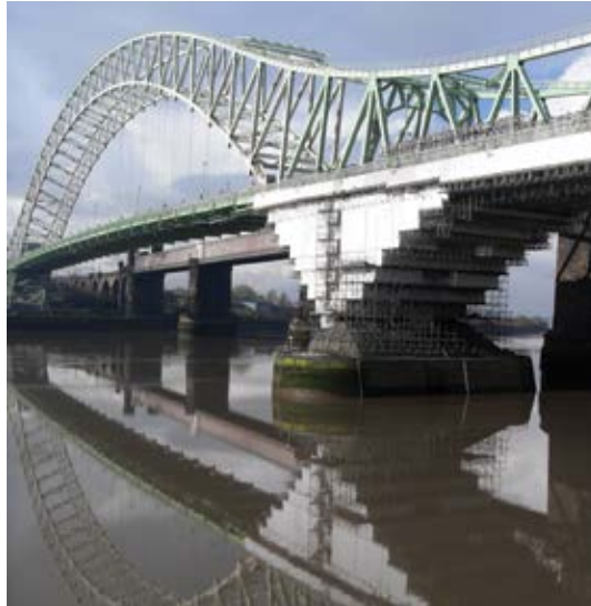
Side view of bridge
