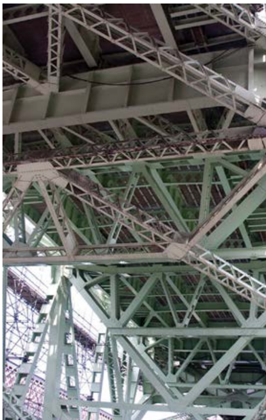
Underside of bridge where "cassettes" were installed
