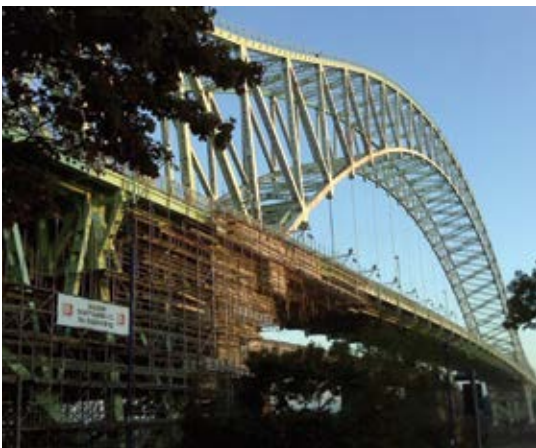
Silver Jubilee Bridge with repair scaffolding in place
