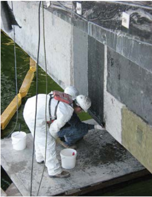
Installation of FRP wrap
