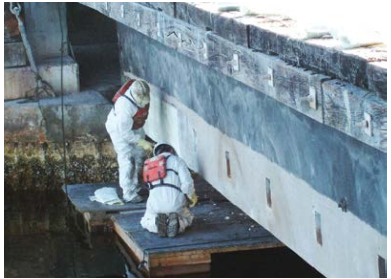
Workers completing repairs on bottom of beams
