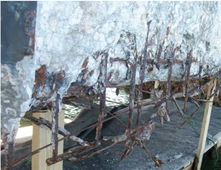
Deteriorated concrete being removed from bottom of beams
