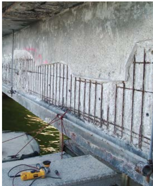
Concrete being prepared for repair on bottom of beams
