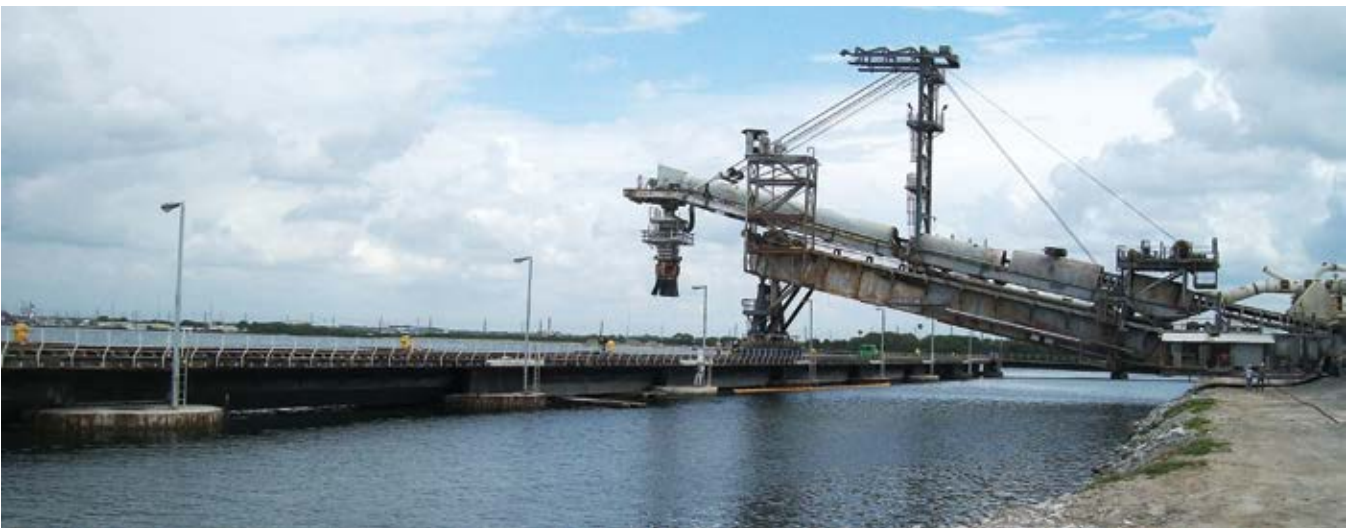
Completed repairs on dock showing loader
