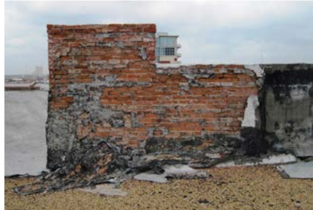
Fig. 2: Roof wall prior to rehabilitation
