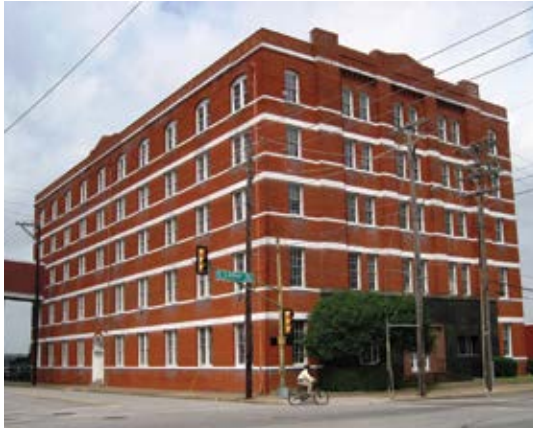
Fig. 1: Building in original condition before "reincarnation"
