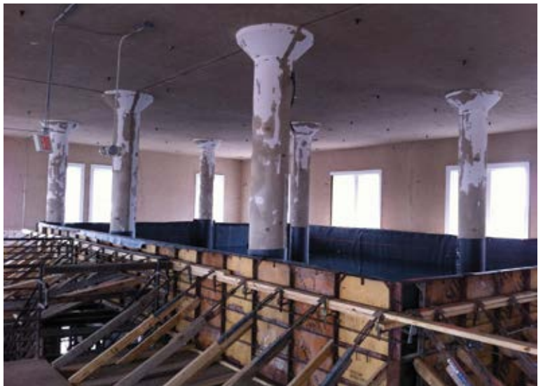
Fig. 4: Load test being performed in accordance with ACI 318-05
