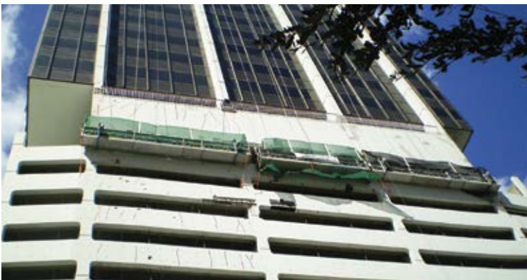
Repairing the south elevation using swing stages
