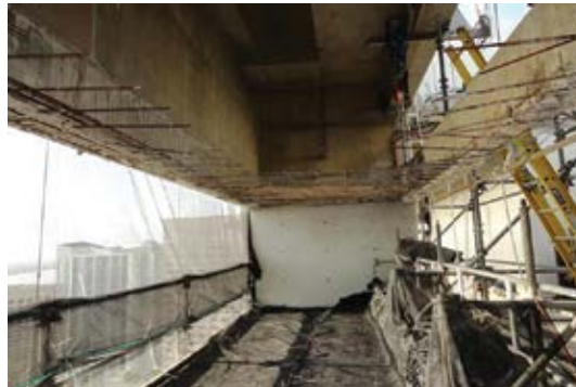
Overhang slab after demolition and “dance floor” with debris protection installed
