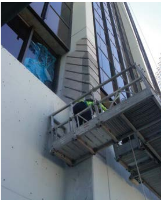
Column build-out and additional reinforcing slots
