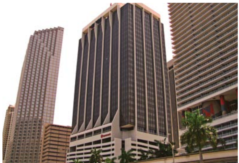
Completed repairs to One Biscayne Tower
