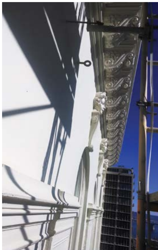
Restoration of architectural details
