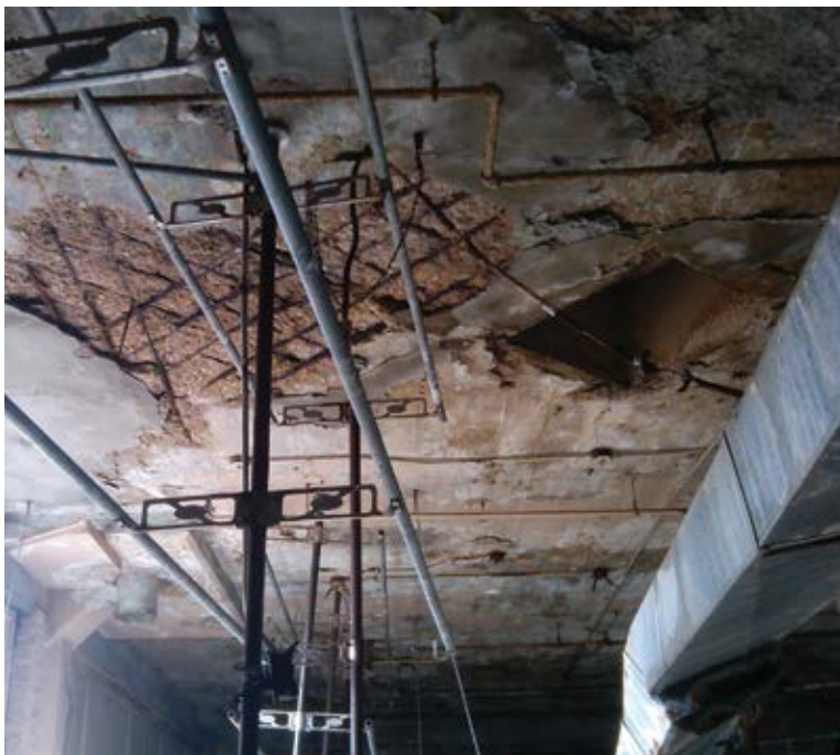
Spalling ceiling
