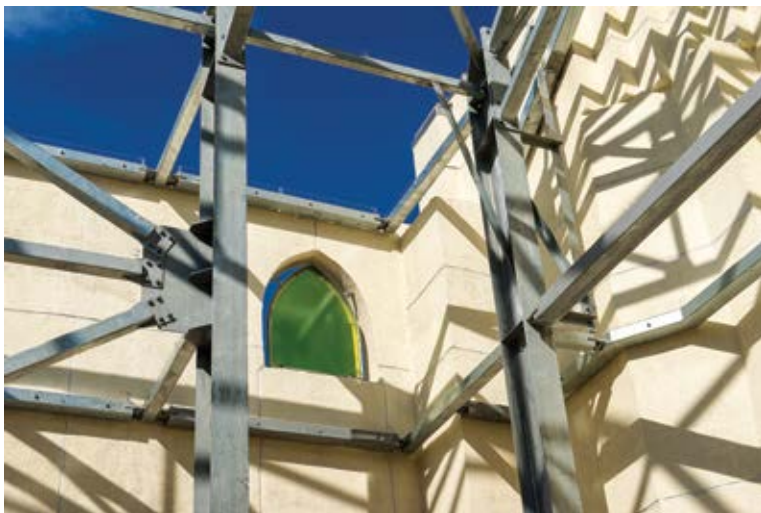
Fig. 7: A cream-colored elastomeric coating brightened the interior finish
