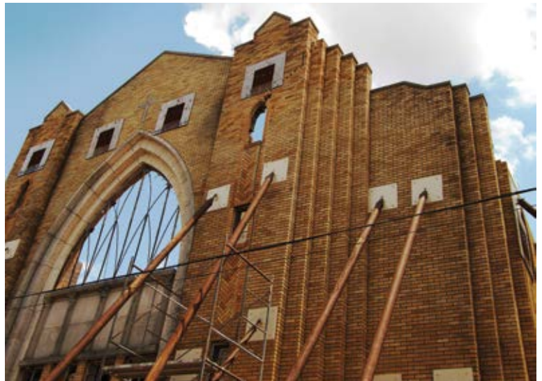
Fig. 4: Emergency shoring and bracing
