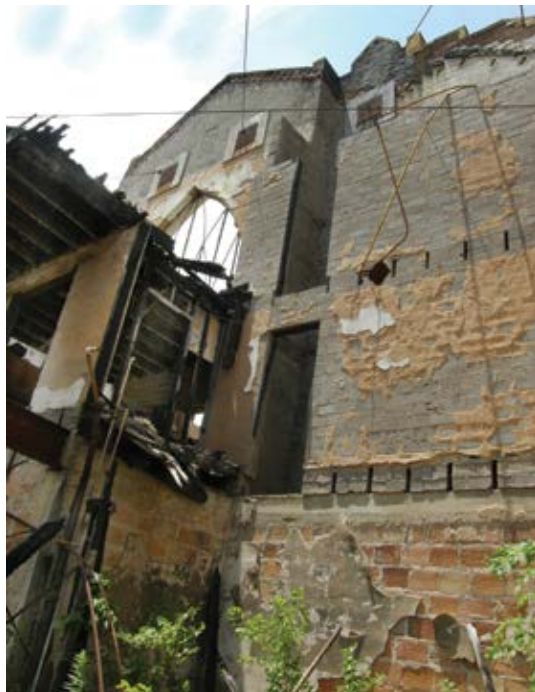
Fig. 1: Masonry wall prior to restoration
