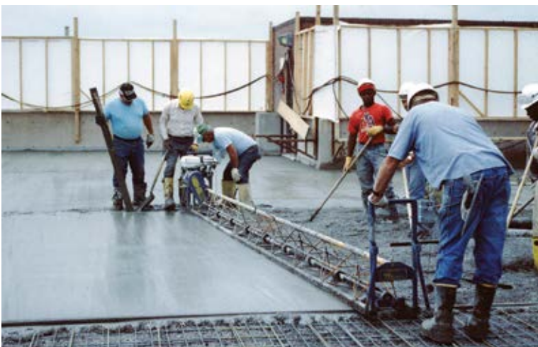
Placement of concrete overlay
