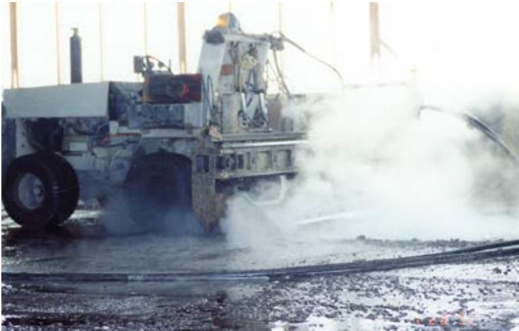
Hydrodemolition in progress
