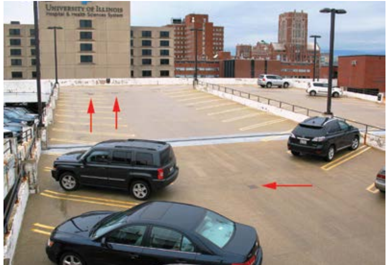
Overlay and localized repairs
