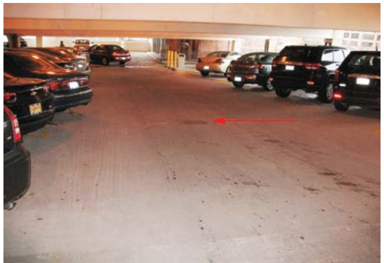
Overlay and localized repairs
