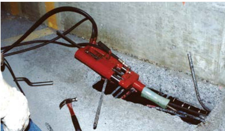
Post-tensioning tendon repair
