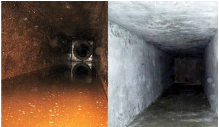
Confined space wall repairs before and after
