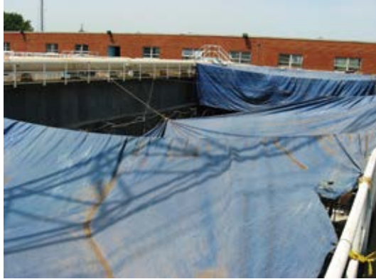
Temporary shading during repair
