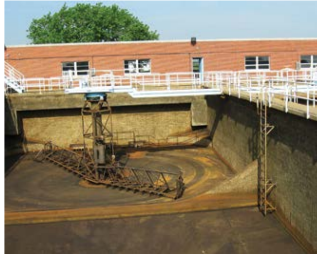
A general view of the original floc/sed basin conditions
