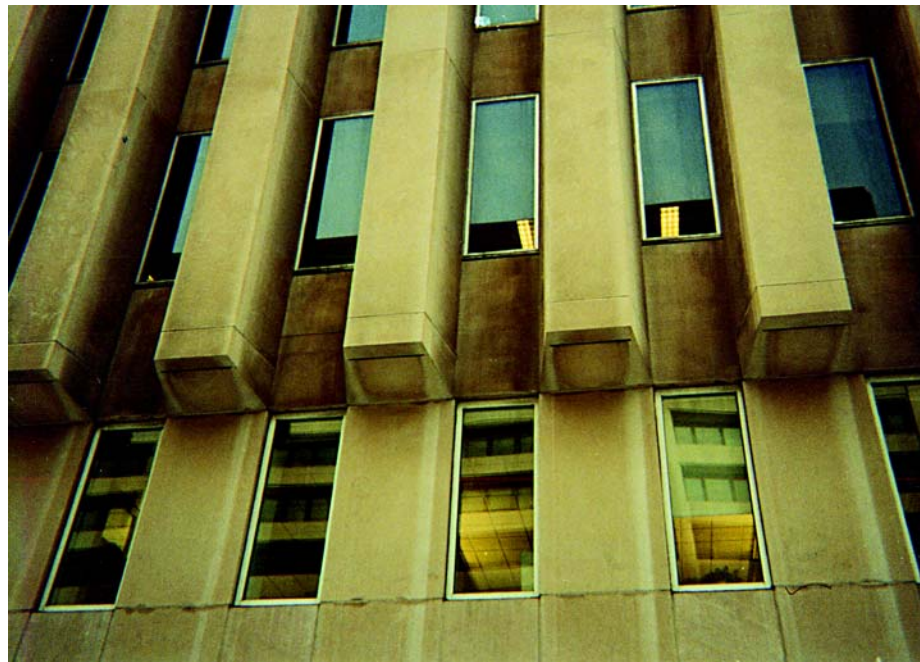
Figure 3: The E Building limestone panels at third floor
