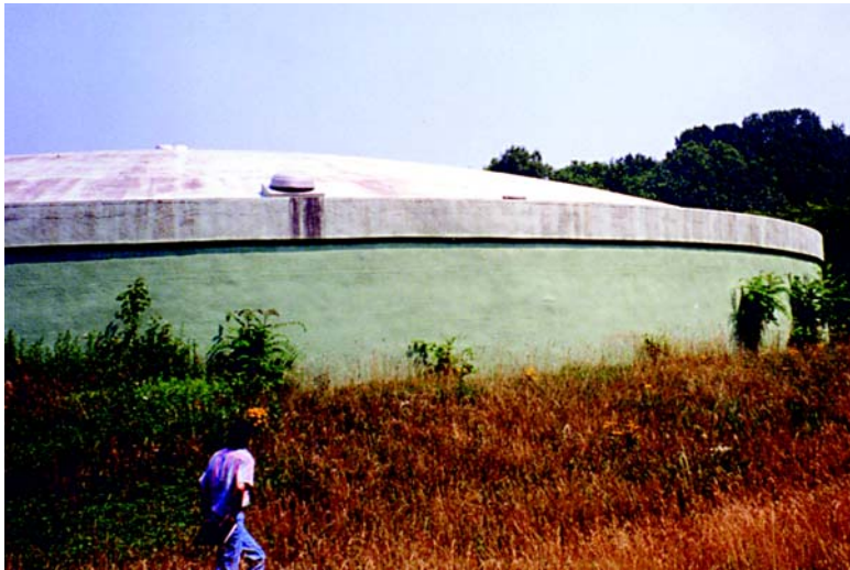
Figure 1: Southside Reservoir before the work
