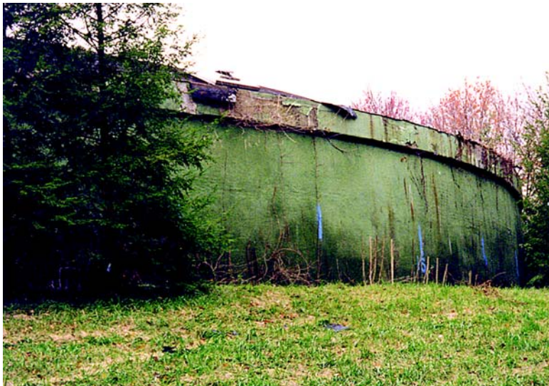
Figure 2: Eastside Reservoir before the work
