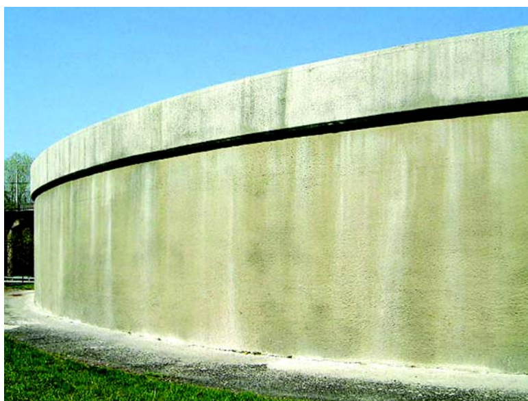
Figure 4: Southside Reservoir after the work
