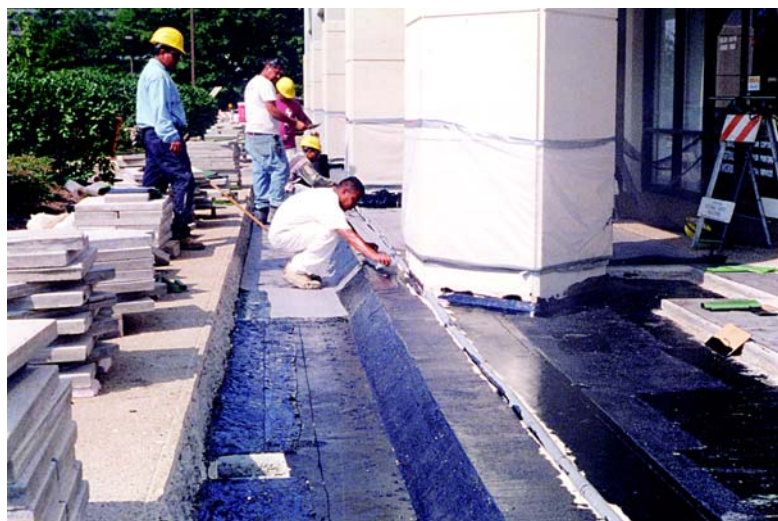
Fig. 6: Ultimately, the building owner may decide to perform spot repairs on the membrane system until the building can be sold or money for complete replacement can be budgeted
