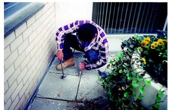
Fig. 2: Test holes should be performed and repaired by a qualified contractor
