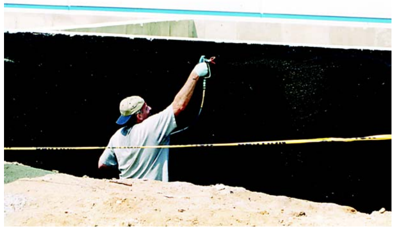
Figure 1: Spray application of cold-applied polymer-modified emulsion
