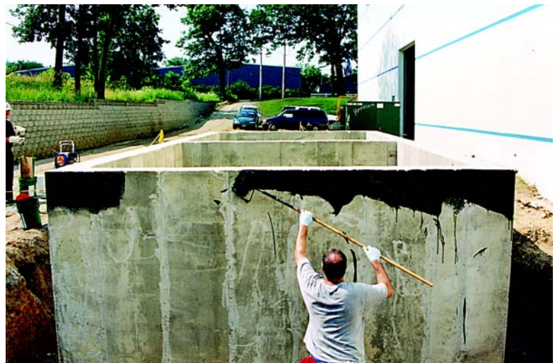
Figure 2: Roller application of cold-applied polymer-modified emulsion
