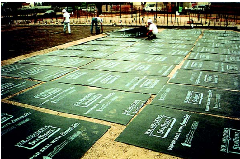
Figure 6: Installation of bituminous vapor barriers
