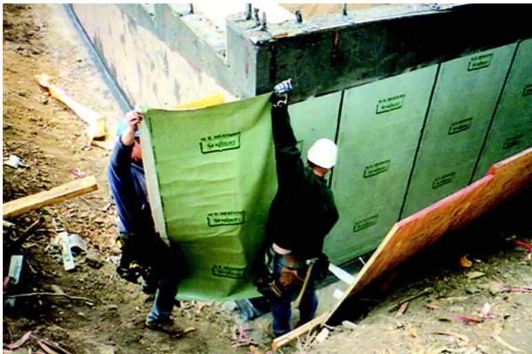
Figure 4: Rubberized asphalt sheet membrane applied to concrete foundation wall
