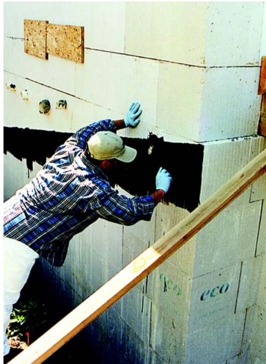
Figure 3: Polymer-modified asphalt emulsion applied on insulated concrete forms
