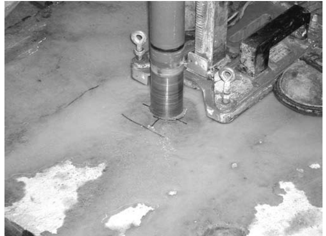
Fig. 10—Coring hole for anode.
