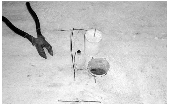
Fig. 11—Secondary hole with reinforcing steel connection.
