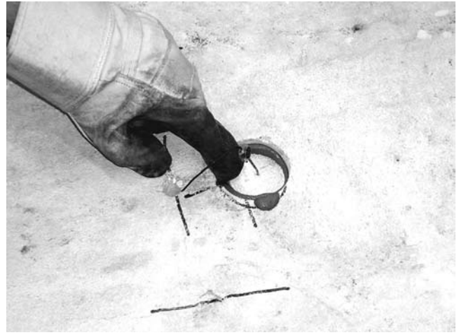
Fig. 13—Anode placed in hole with patching material.
