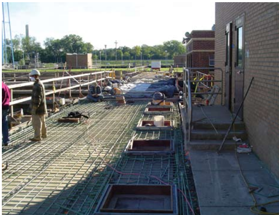
During construction (forming and steel placement for new slab)
