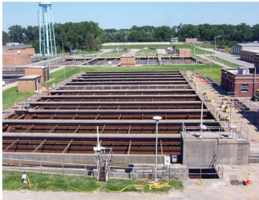
Overall existing project before reconstruction
