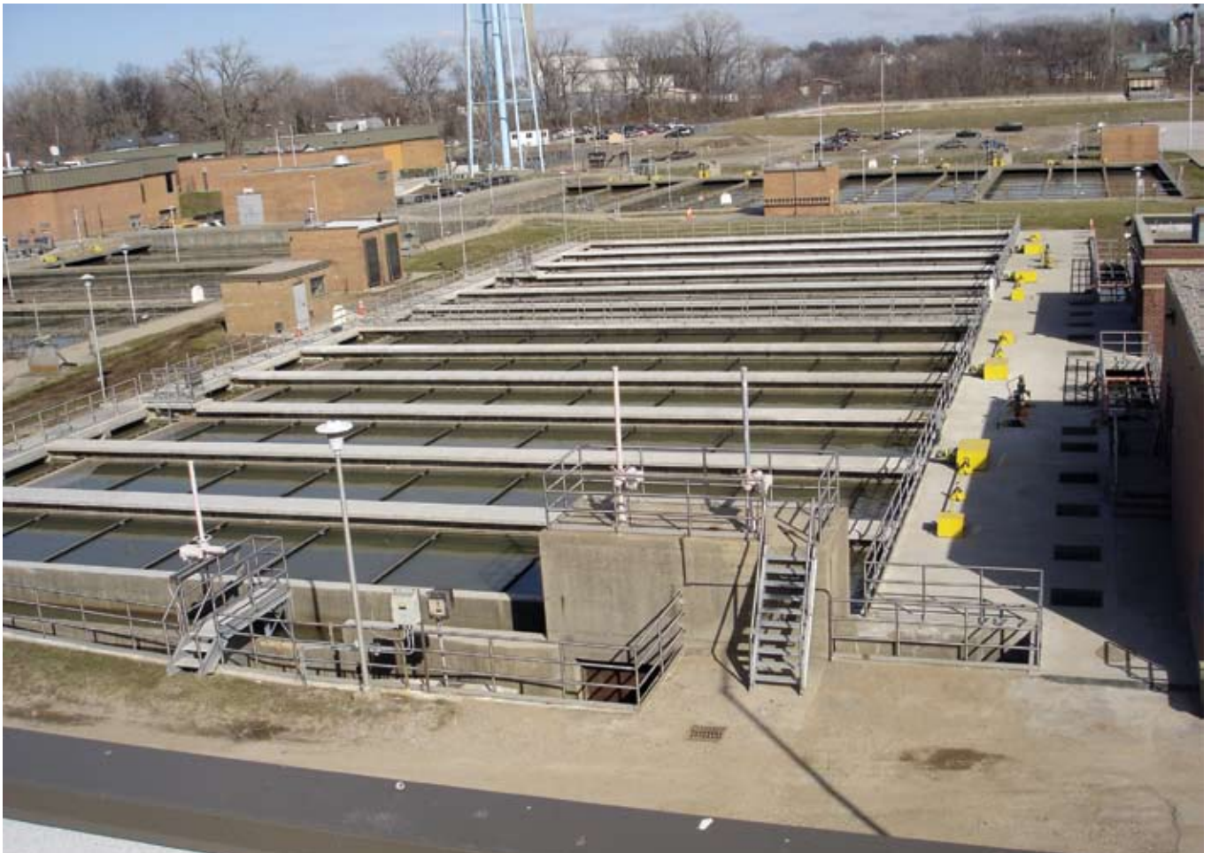
Overall completed project
