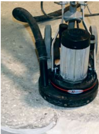
Coatings removal using a floor grinder
