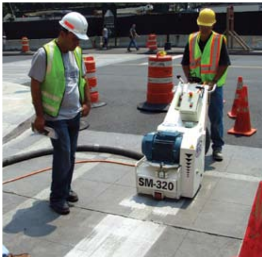
Concrete shaver cutting grooves in Manhattan sidewalk
