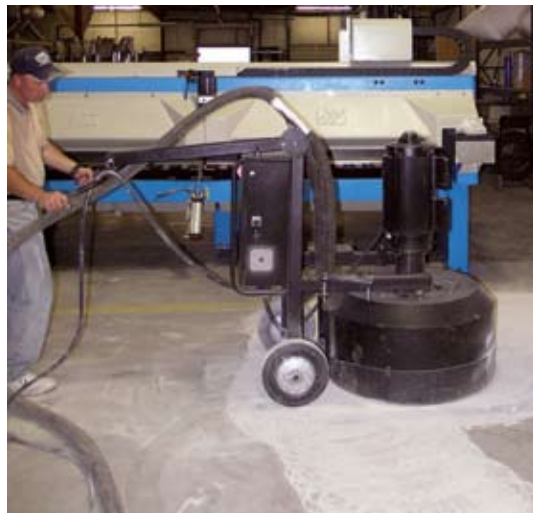
First step of the concrete polishing process
