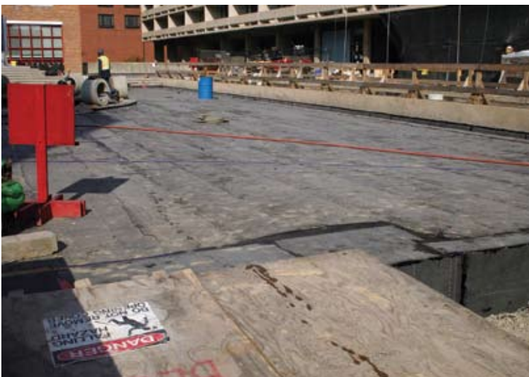
Lower level after new hot-applied waterproofing system was installed
