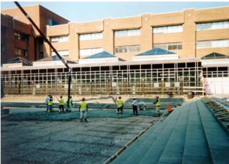
Lower level—placement of lightweight concrete fill
