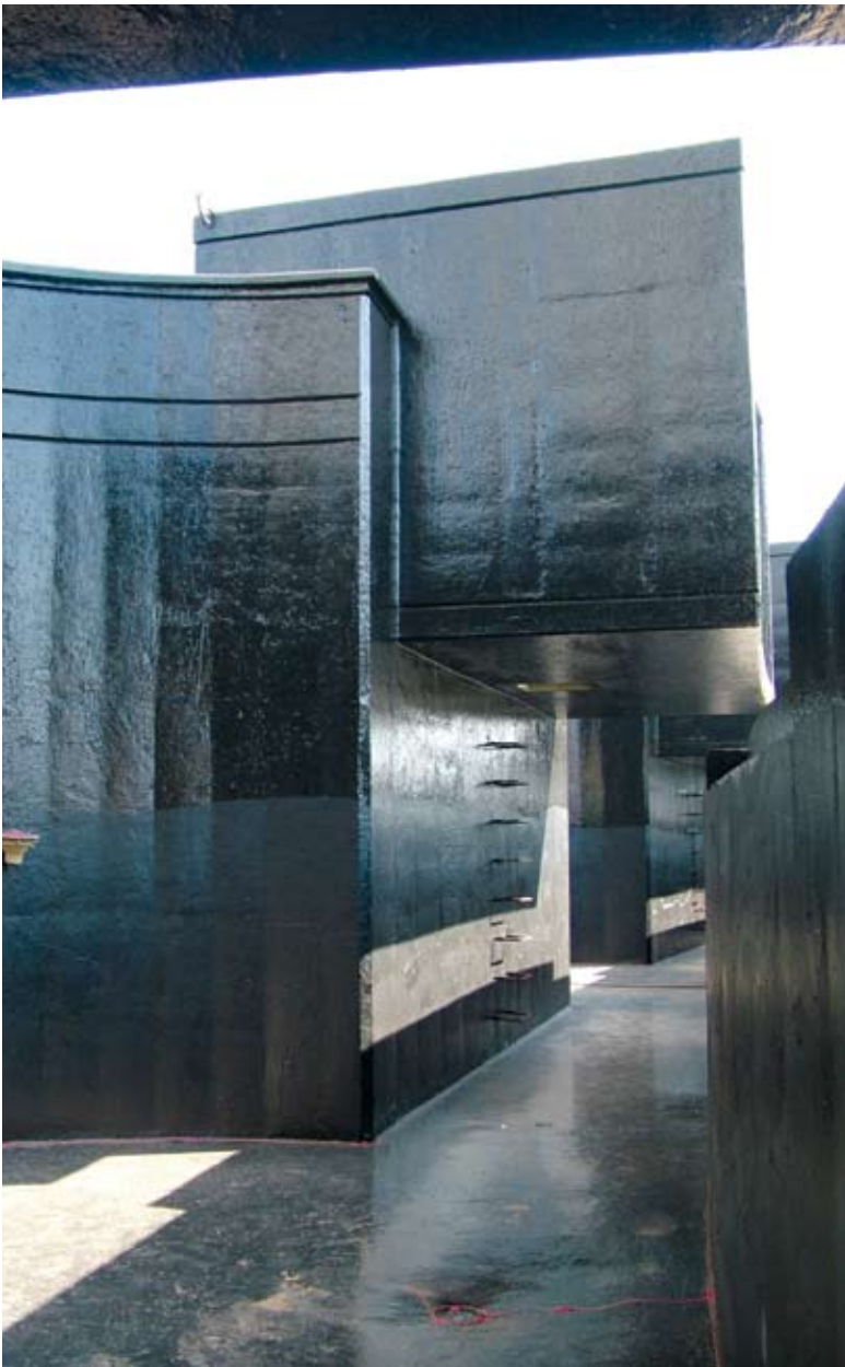
Main fountain: completed waterproofing membrane system in the lower pool area
