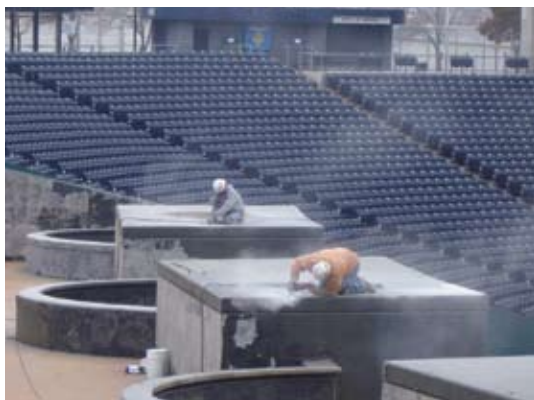
Removal of existing coatings
