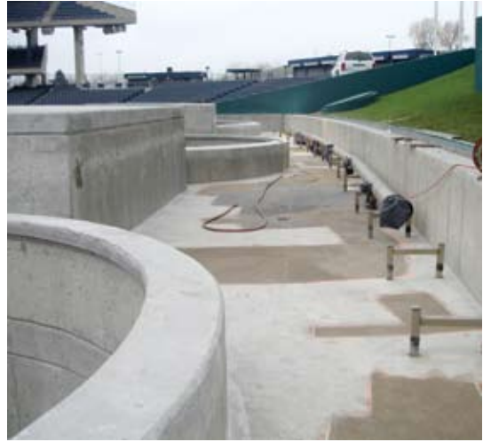
Secondary fountain: completed concrete slab repairs
