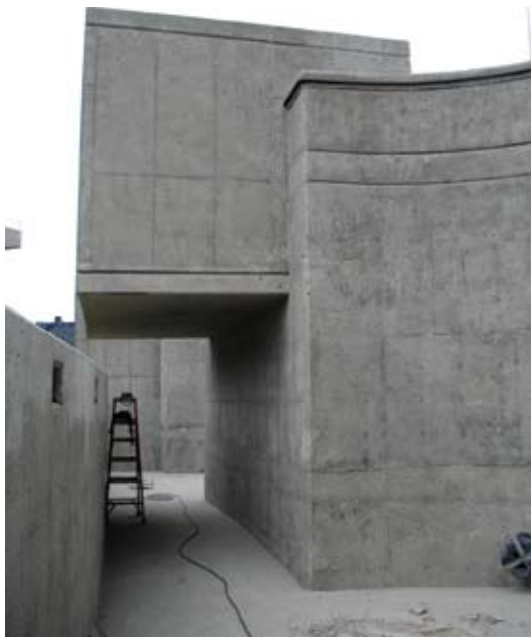
Lower pool area: main fountain after coating removal
