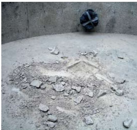
Concrete slab delamination removal
