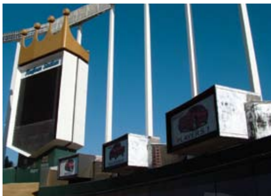
Removal of existing coatings at the signage boards
