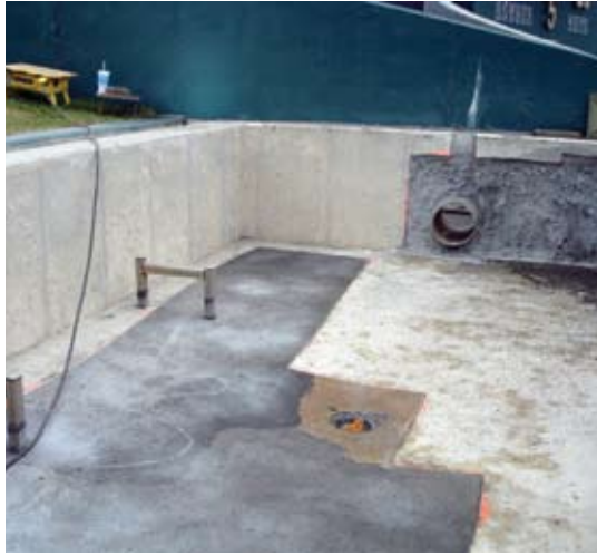
Completed concrete slab repairs
