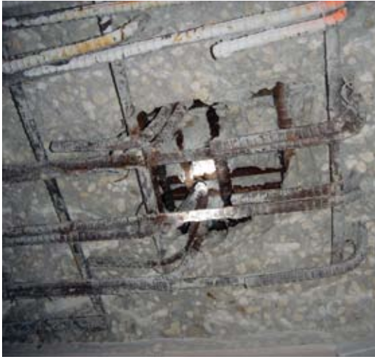
Fig. 7: Concrete and reinforcing steel being prepared for repair
