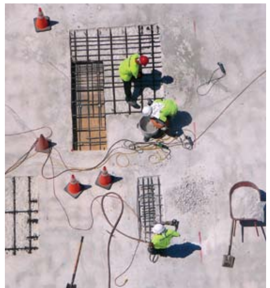
Fig. 2: Workers performing the concrete repairs
