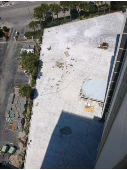
Fig. 3: Work Area "A" test site as seen from roof of building
