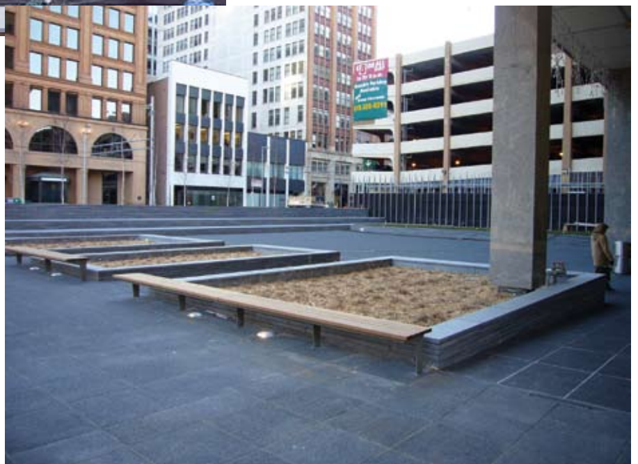
The completed plaza before landscaping was installed
