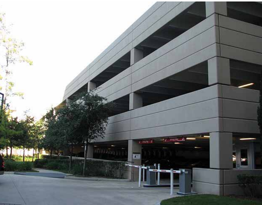
Fig. 5: Woodlands Waterway Marriott Parking Garage
