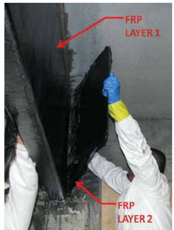
Fig. 4: (a) Schematic plan view of end of double-tee stem showing FRP layers; and (b) installation of FRP Layer 2
