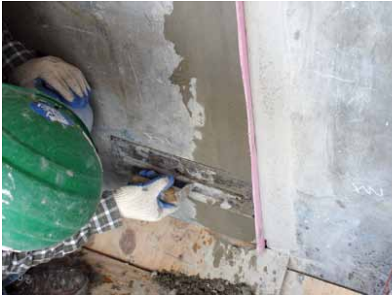
In-place mockup of repair materials being conducted
