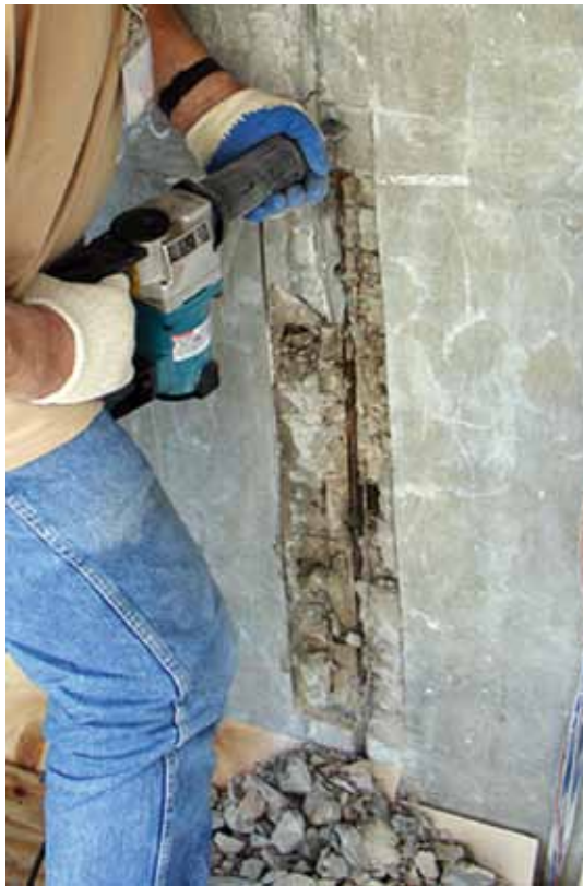
Demolition for in-place mockup
