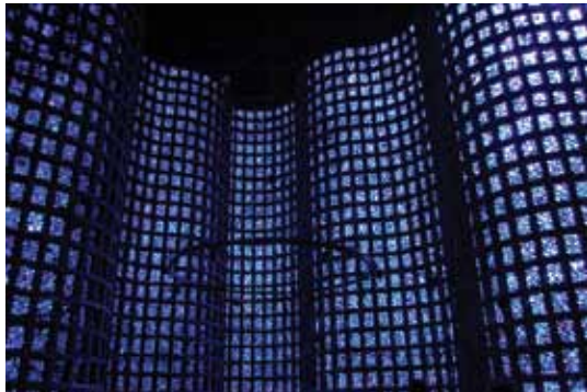
The building technique known as "dalle de verre" allows the light to shine through the cobalt blue pieces of glass, offering visitors the feeling of floating through space
