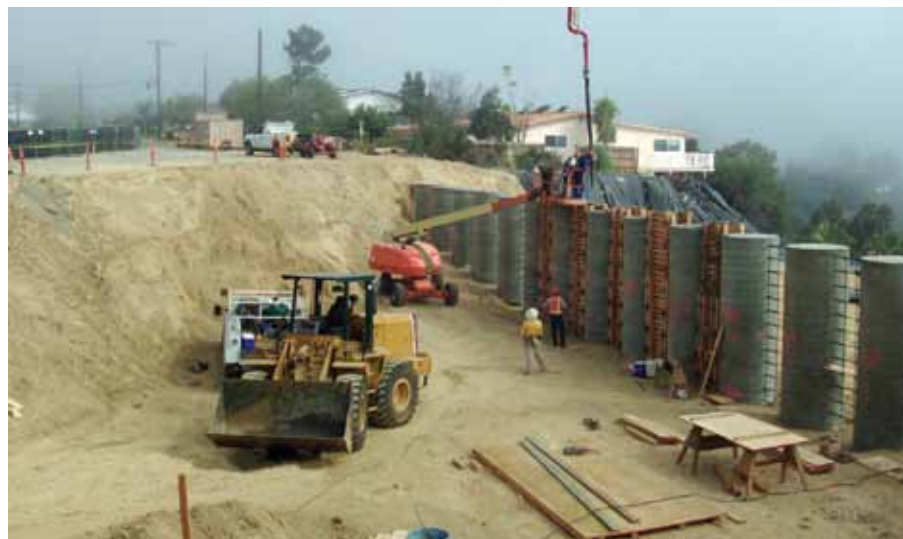
East-side shoring panel wall construction
