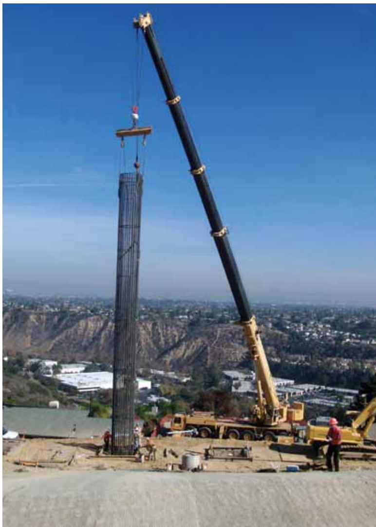
Setting of reinforcement cage using 500 ton (453.6 metric ton) crane
