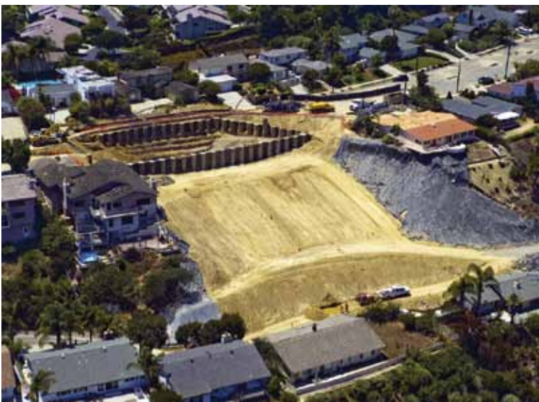
Aerial view of shoring during repairs
