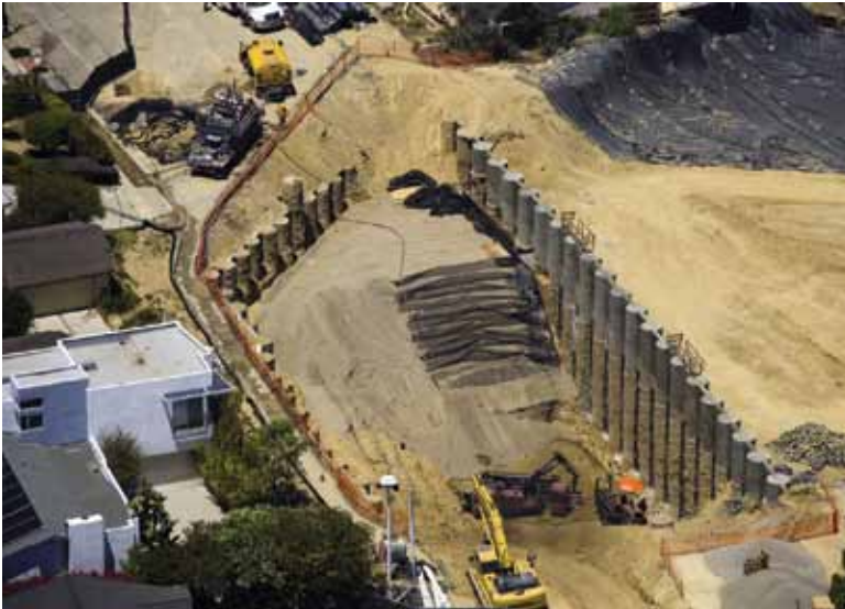
Geogrid reinforced fill in Slot 1 excavation
