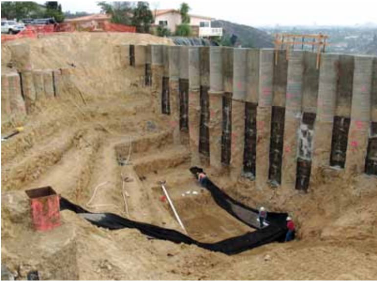
Temporary and east-side shoring during excavation
