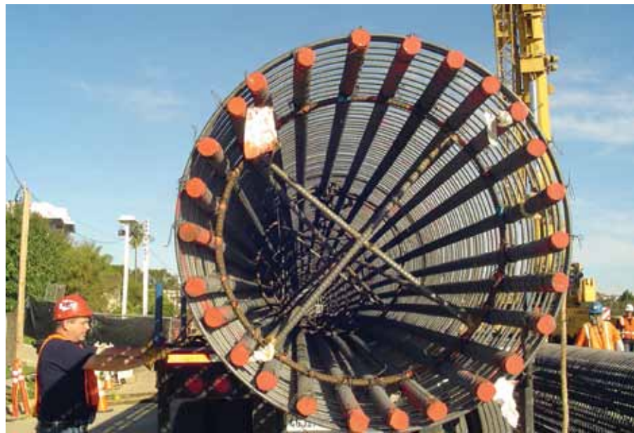
Closeup of reinforcement cage
