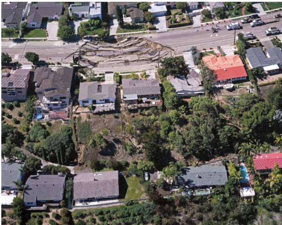
Soledad Mountain Road landslide, October 3, 2007
