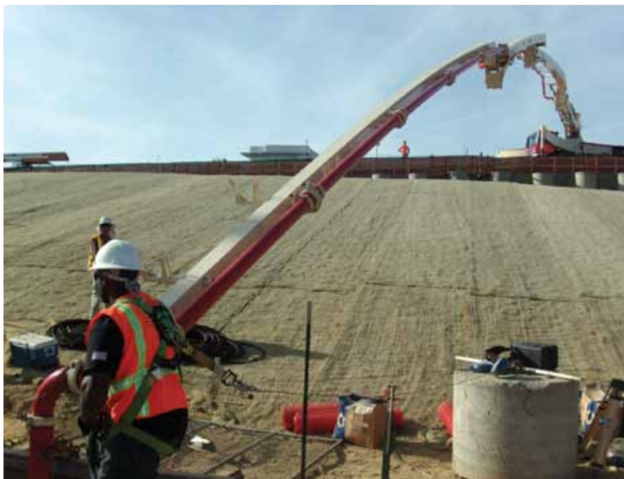
Pumping concrete using 170.6 ft (52 m) boom truck
