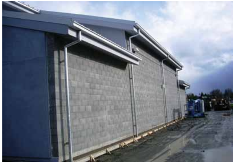
Fig. 1: Exterior view of the CMU wall
