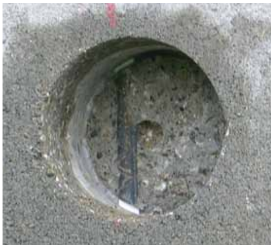
Fig. 7: Partial depth core showing good bond around the reinforcing steel
