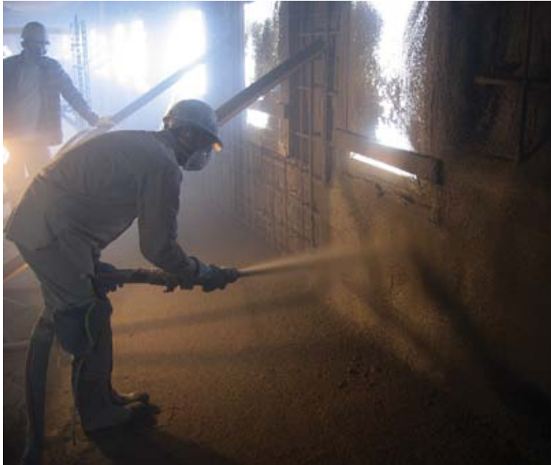
Fig. 5: Shotcrete backup wall fastened to the restored brick masonry veneer
