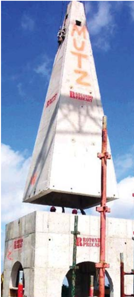
Fig. 3: Precast concrete for bell tower backup wall
