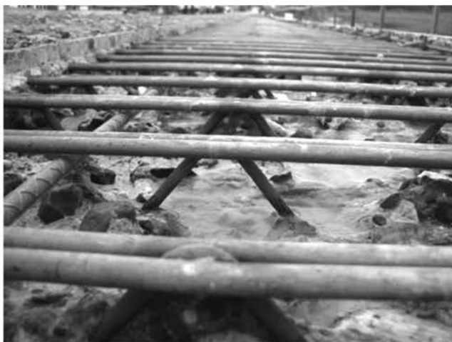
Fig. 3—Reinforcing steel and bar joist top chords exposed using hydrodemolition.
