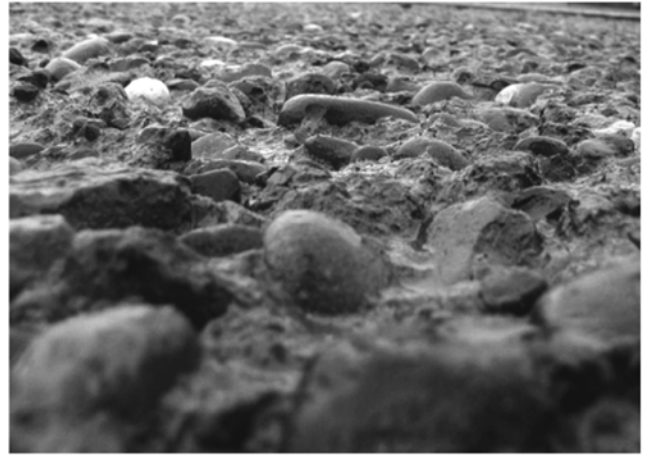
Fig. 1—Surface profile after hydrodemolition.
