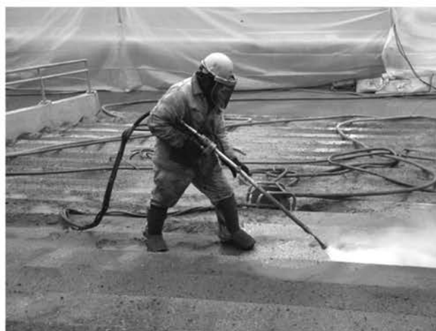
Fig. 7—Hand lance for hand-held hydrodemolition
