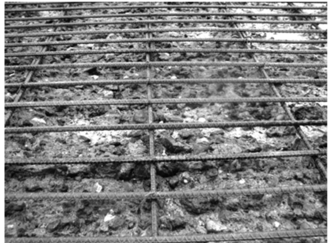
Fig. 2—Reinforcing steel exposed using hydrodemolition.
