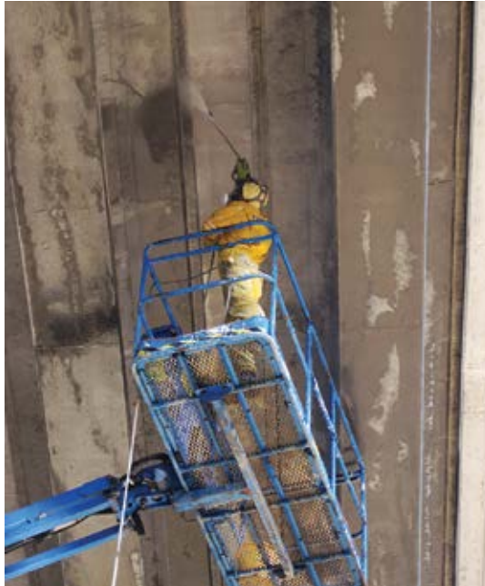
Fig. 6: Overhead airless spray application of a pure silane
