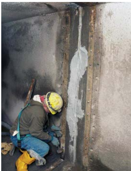
Fig. 9: Construction joint repair after removal of rubber seal
