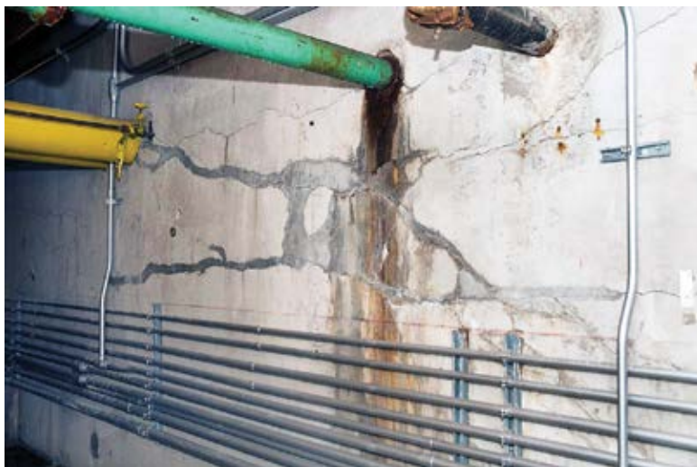
Fig. 2: Crack gauges installed at cracks in pedestrian tunnel
