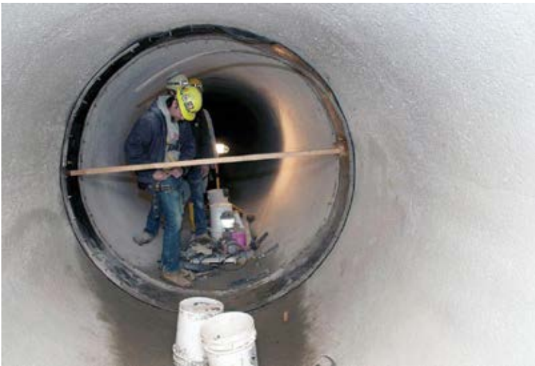
Fig. 10: Installation of new EPDM seal in conduit
