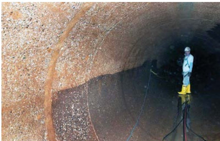
Fig. 8: Surface preparation within conduit
