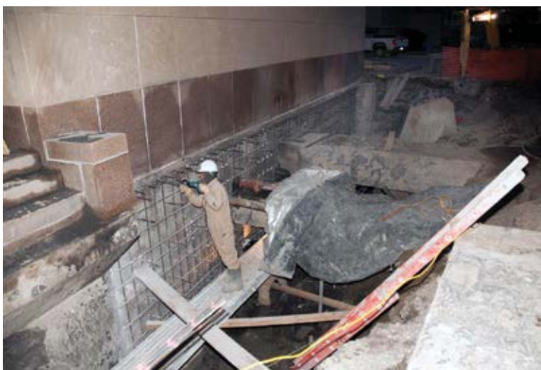
Fig. 6: Installation of reinforcing steel in new wall at pedestrian tunnel
