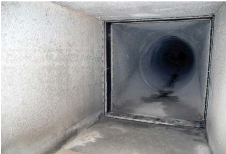
Fig. 5: Completed conduit following leak repair and installation of waterproofing agent
