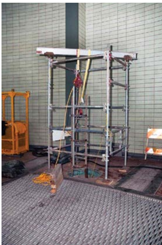
Fig. 1: Access to raw-water conduit for manned entry inspection
