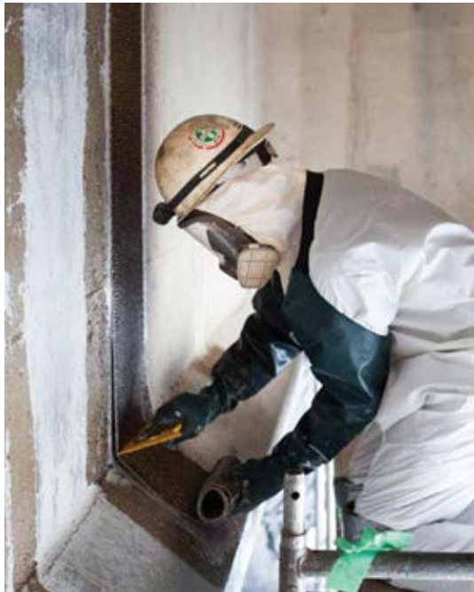
Fig. 4: Installation of saturating resin and carbon fiber wrap
