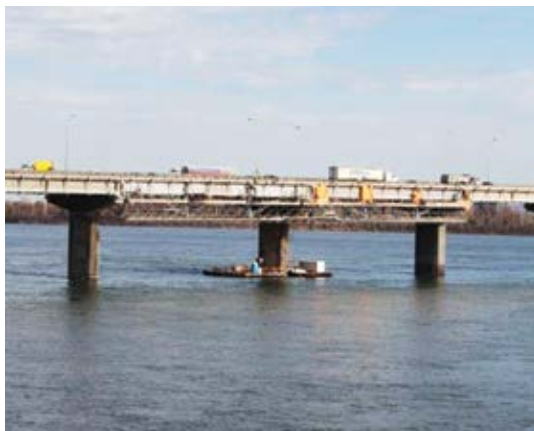
Fig. 6: View of the suspended scaffolding setup
