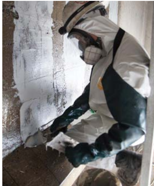
Fig. 3: Application of epoxy paste
