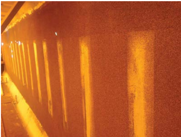
Fig. 5: CFRP with sand broadcast
