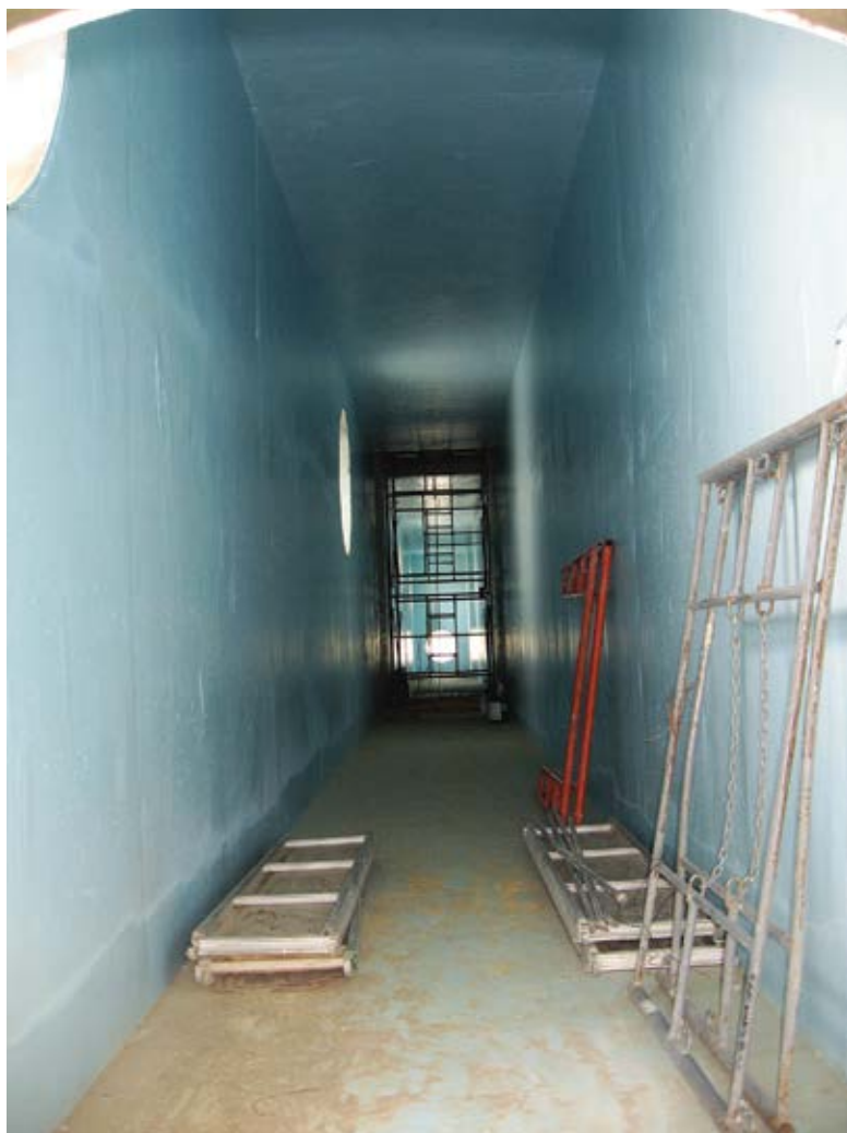
Fig. 5: Epoxy-based liner applied to surface of a wastewater effluent channel
