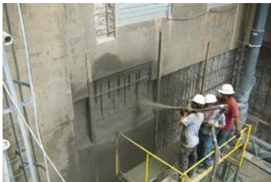
Fig. 3: Installation of spray-applied repair mortar at vertical repair areas
