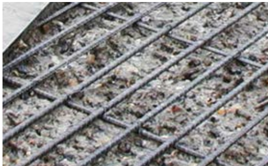
Fig. 2: Hydrodemolition can expose and clean reinforcing steel
