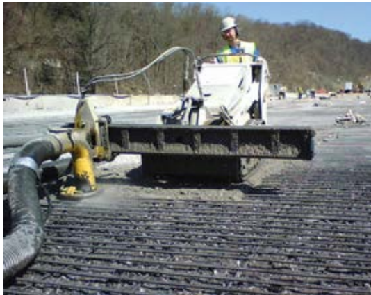
Fig. 5: Small track unit used to vacuum debris
